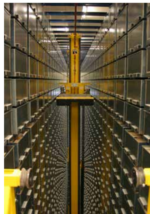
THE AUTOMATED STORAGE AND RETRIEVAL SYSTEM WAS INTRODUCED AT THE IRVING K. BARBER LEARNING CENTRE IN 2009.
